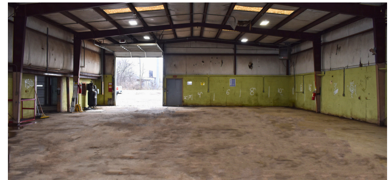
Clear Span in Half of Building
